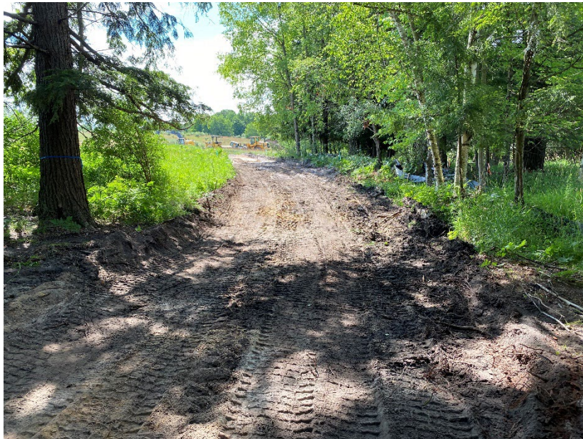
Trail rough grading at box culvert crossing
