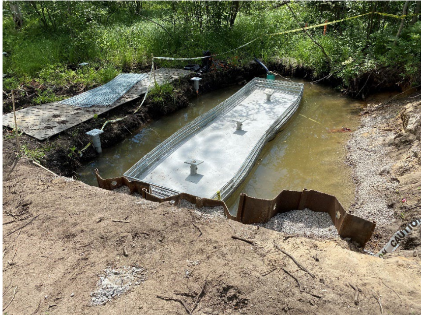
Acme Creek Crossing western boardwalk abutment (partially constructed)
