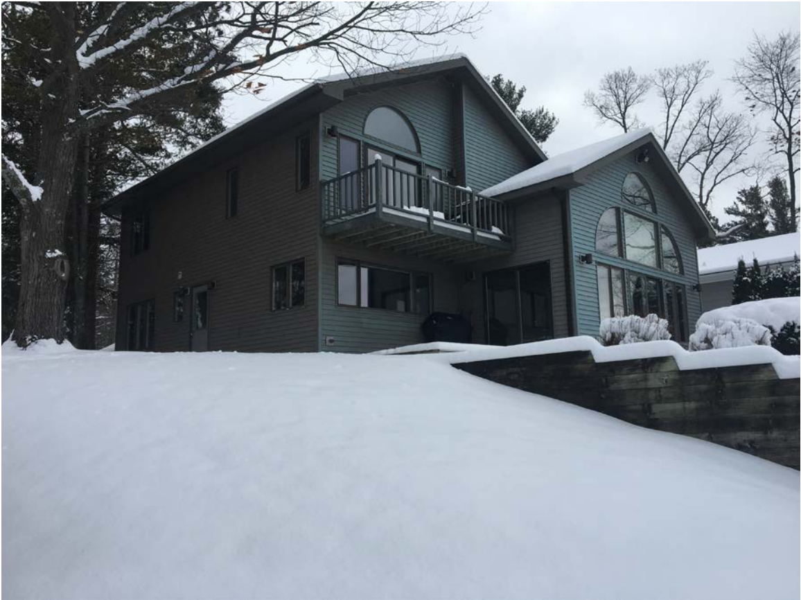
Photo 1 – North elevation where addition is to be added
