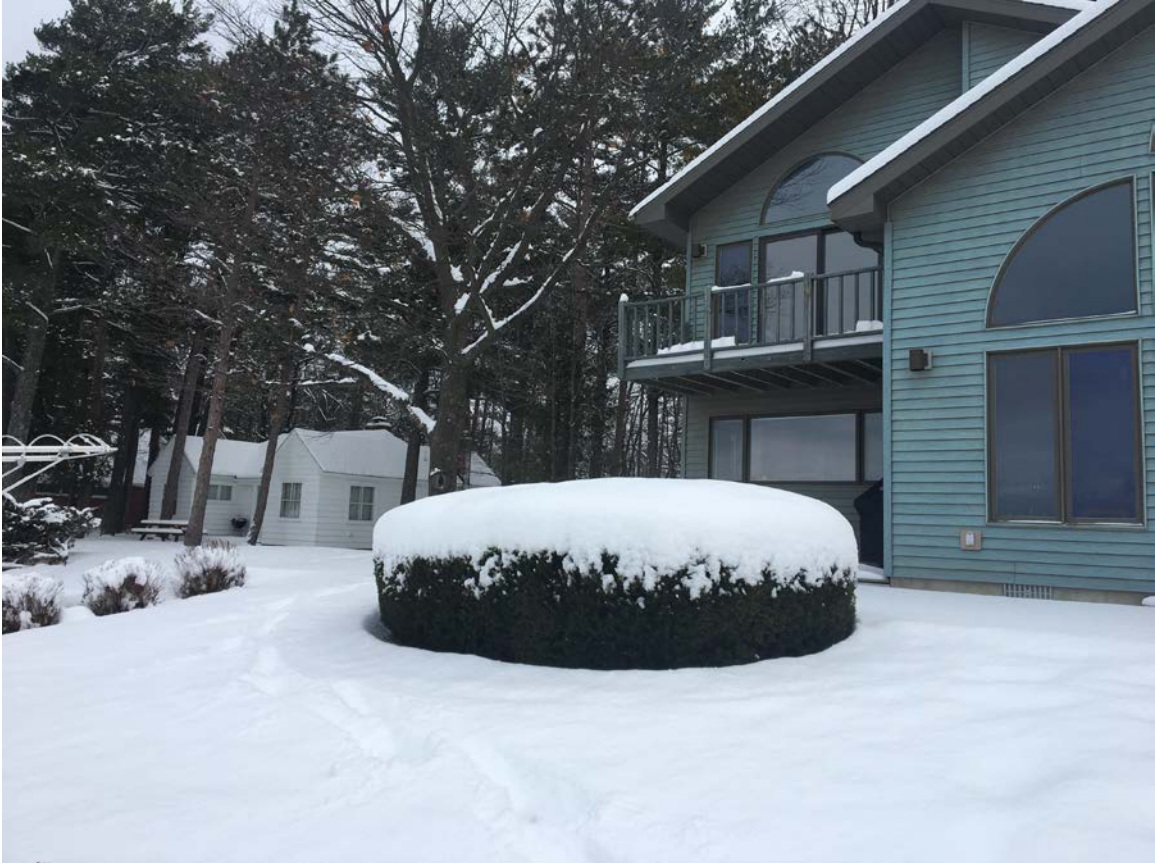
Photo 4 - East elevation, waterfront side
