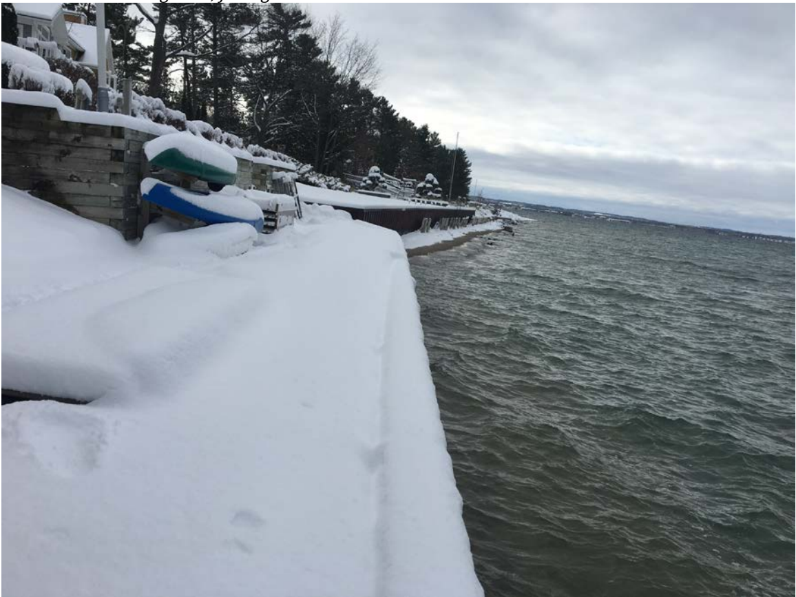
Photo 2 – Retaining wall, facing south
