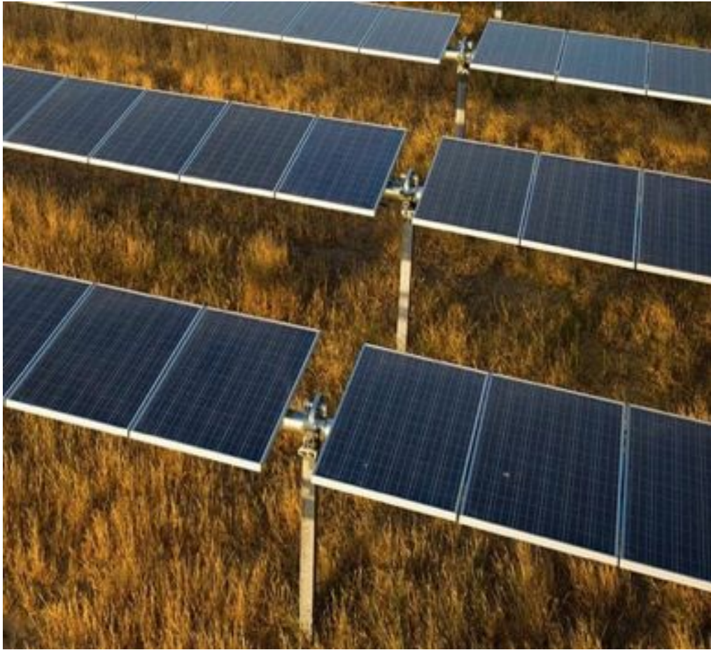
Typical configuration of single-axis solar array.
