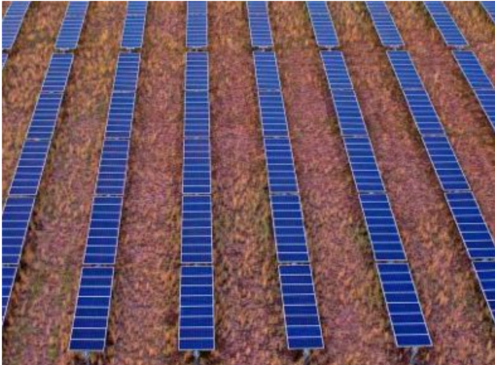
Typical configuration of single-axis solar array.
